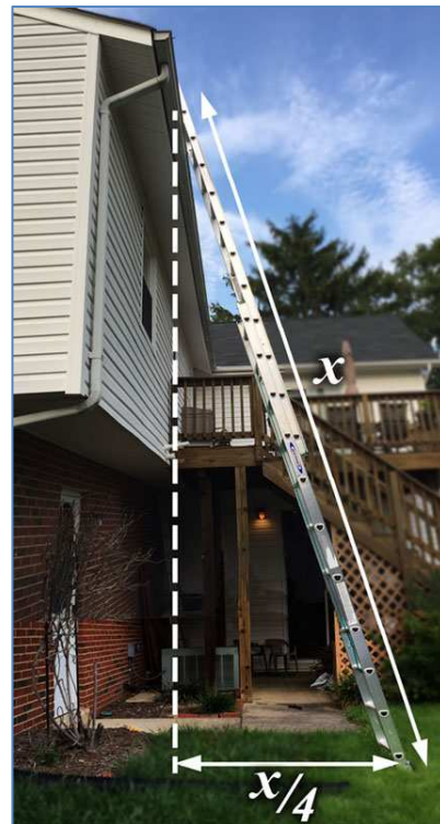
Figure 8. The distance from the base of the ladder to the structure
