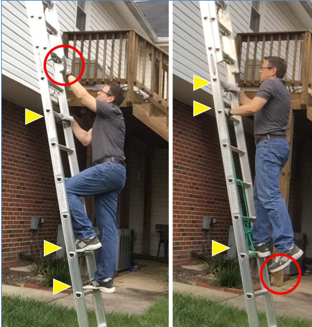
Figure 9. Maintaining three points of contact at all times
