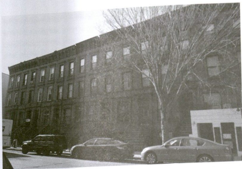
04.C Typical low-rise housing in Harlem.
