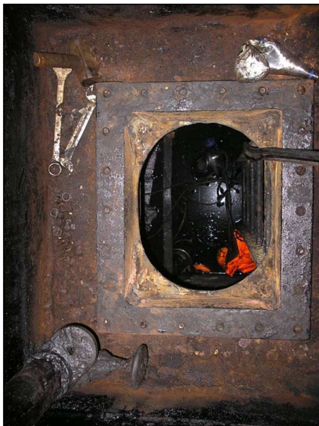
No.4 port outer double bottom tank manhole
